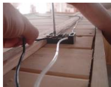
FIG-18 outer line on top board
