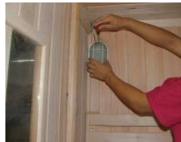
FIG-20 install the glass cover
