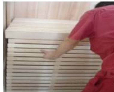
FIG-12 Assemble the left long sitting baffle
