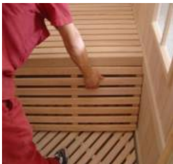
FIG-13 Assembling right short baffle
