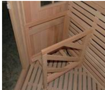
FIG-24 disassemble the wooden frame
