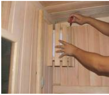
FIG-21 install the wooden cover
