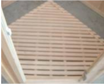
FIG-9 place the floor board
