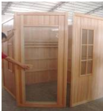
FIG-7 Assembling the front board
