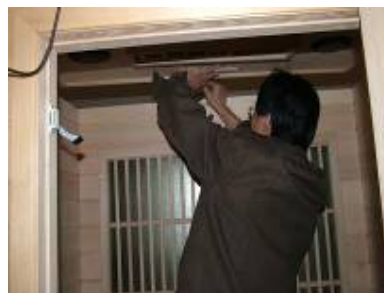
FIG-13 Leading the wires of heaters onto the board through the corresponding hole
