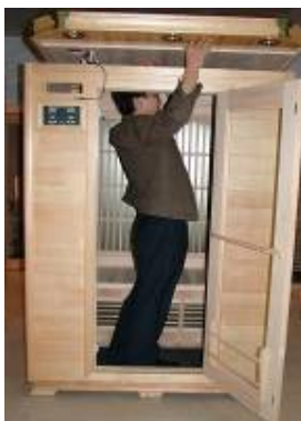
FIG-12 Setting the top board
