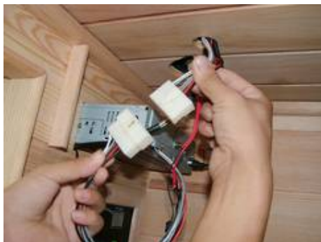
FIG-17 Link the CD connectors
