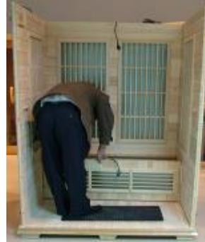
FIG-8 Assembling sitting board's support
