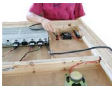
FIG-15 Put down the wires into the sauna cabin
